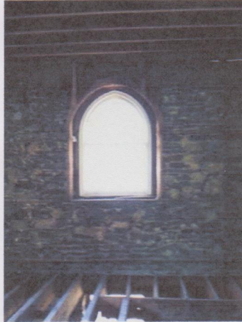
Existing Side windows- clear glazing
