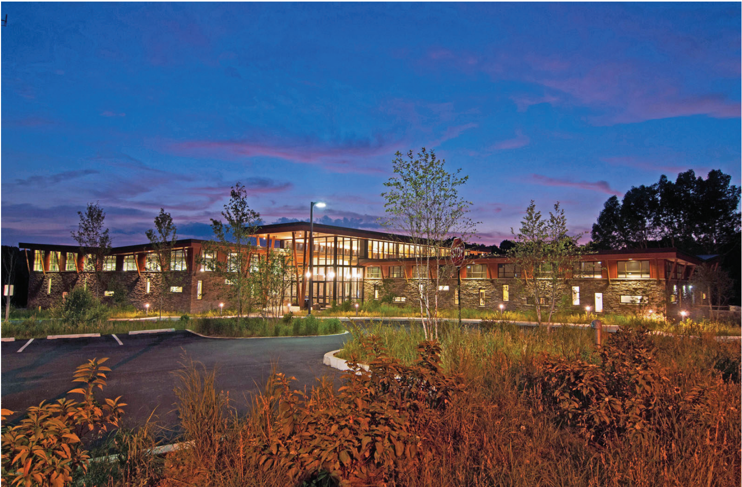
Haverford Township Community Recreation & Environmental Center in Havertown, PA (Kimmel Bogrette Architecture)
